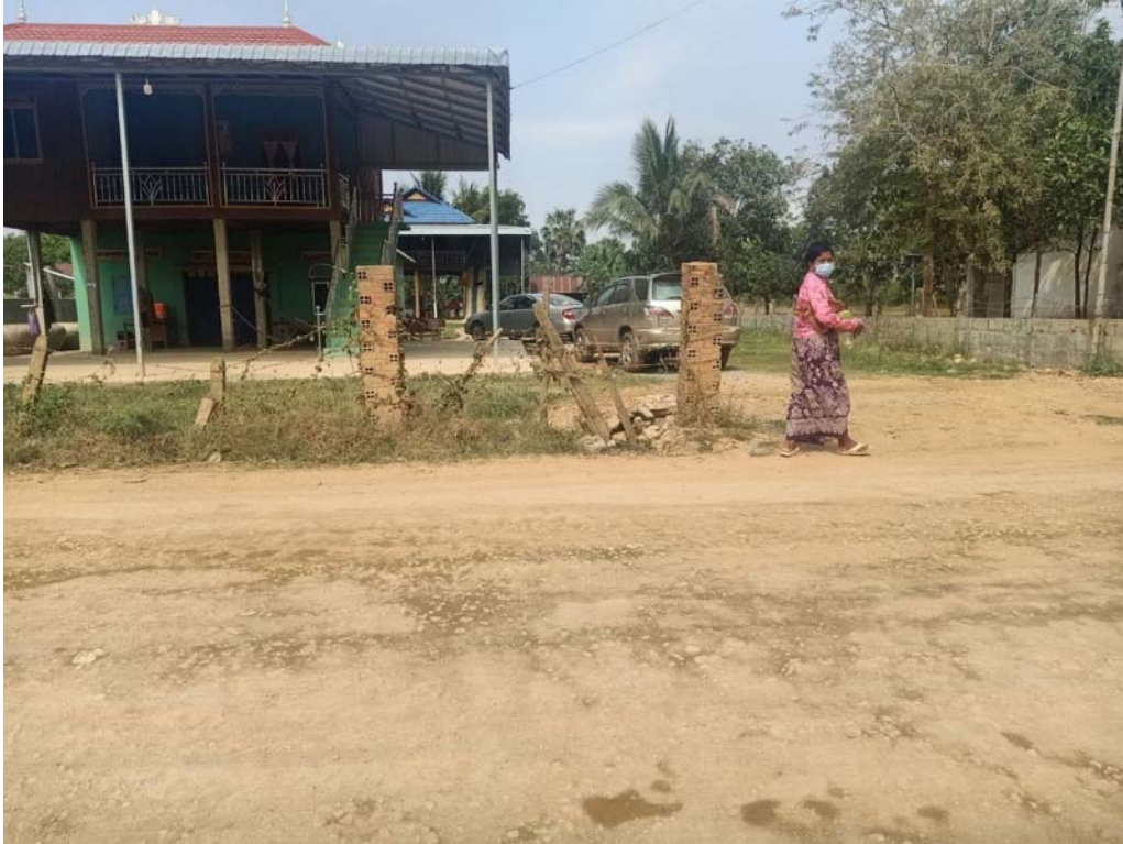
Front Gate Columns owned by Ms. So Varpp, she agreed to remove her front gate columns herself and agreed to get 300,000 Riels
