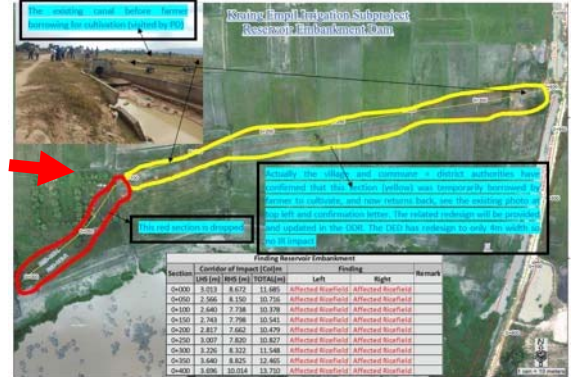
Annex 7: Drone image of Kraing Empil reservoir embankment (PK 0+000 to PK 0+400)
