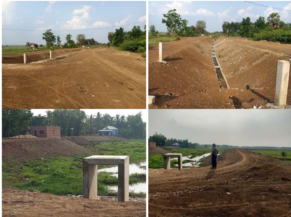
Toul Pring irrigation subproject (Photo taking in April 2022)
