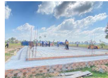
Figure II-2: AC Warehouse construction work progress
