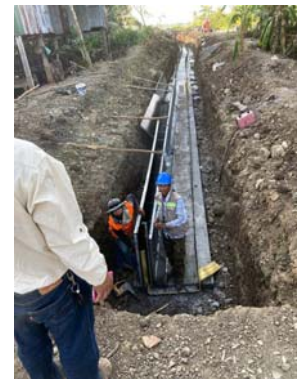
Figure II-1: MoWRAM construction work progress
