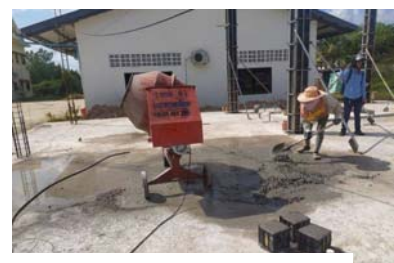
Figure II-23: The construction of the Training building is in progress
