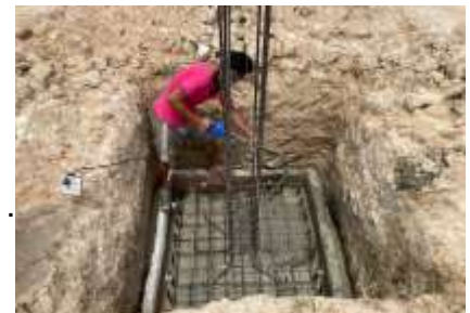
Figure 3: AC Warehouse construction work progress
