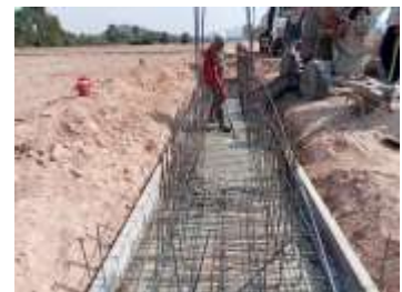
Figure 1: MoWRAM construction work progress
